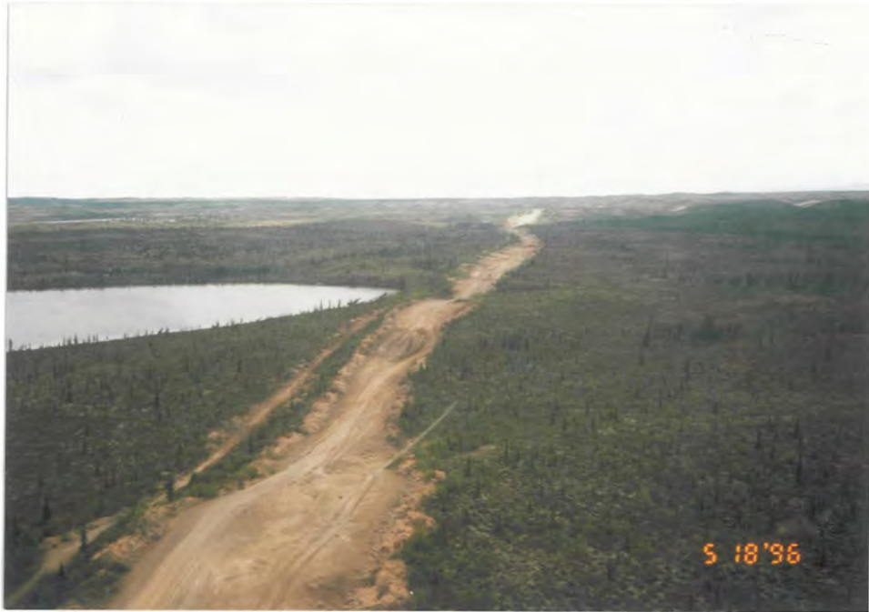
Photo 1. ILIAMNA-NONDALTON ROAD - May 18, 1996. Expanded footprint. Increased off-road activity due to substandard roadbase.
