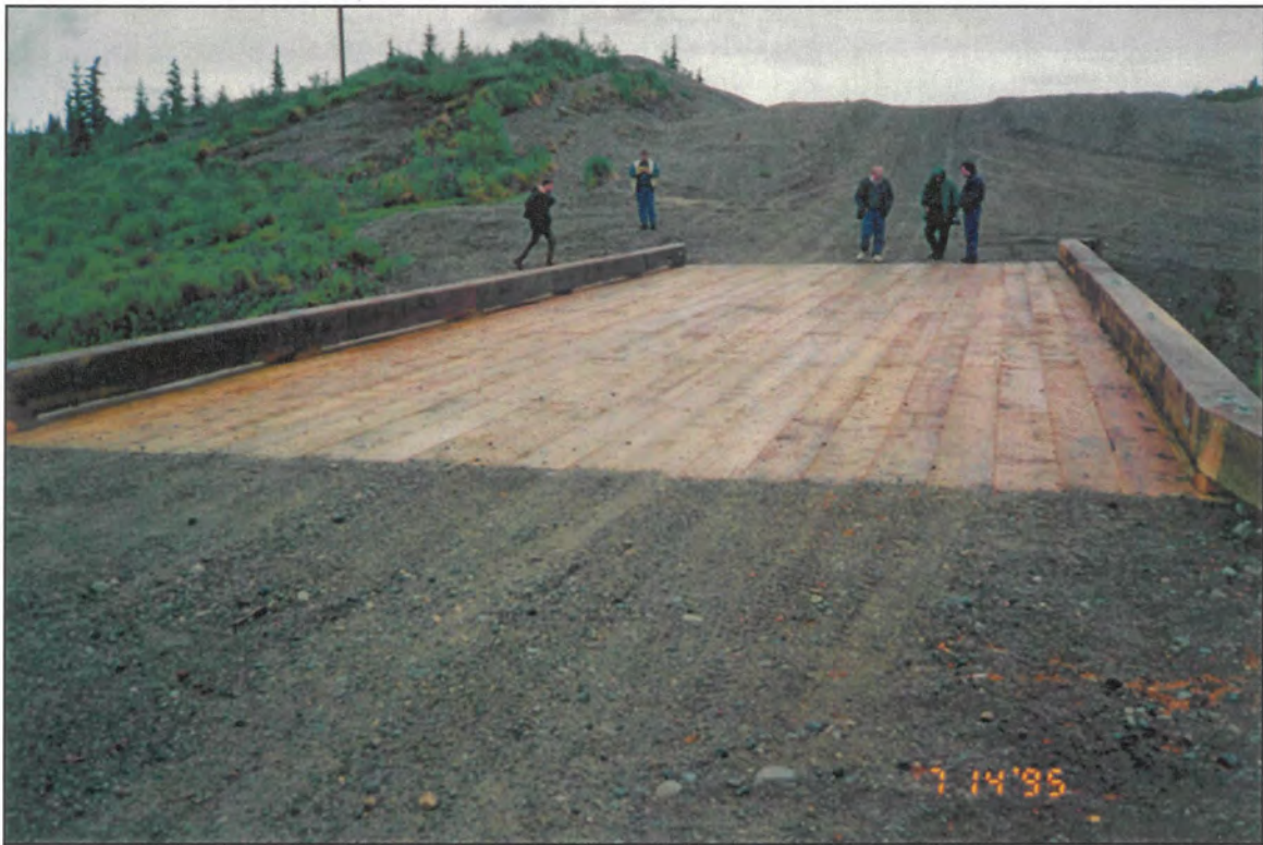
Photo 3: Alexcy Creek Bridge, reconstructed in 1995. 7-14-95.
