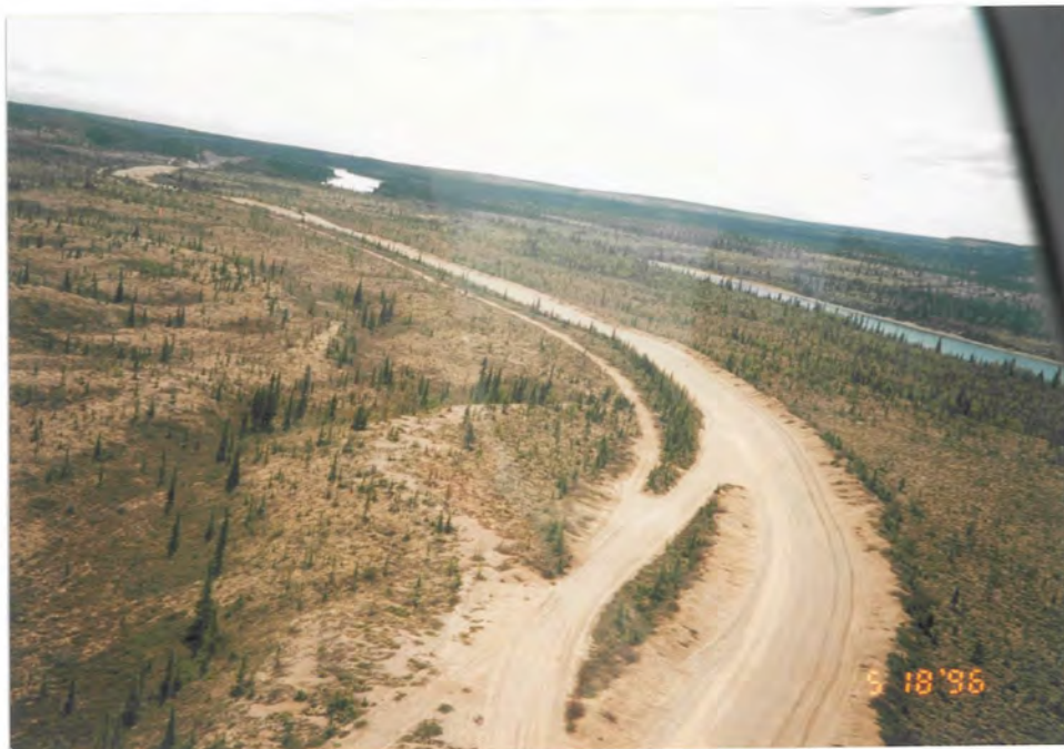
Photo 2. ILIAMNA-NONDALTON ROAD - May 18, 1996. Expanded footprint. Increased off-road activity due to substandard roadbase.
