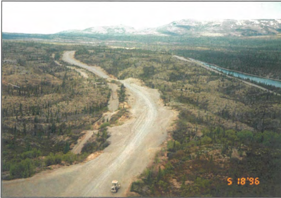
Photo 11: Aerial view of wide footprint along the Iliamna-Nondalton Road. Looking south towards Iliamna. 5-18-96.
