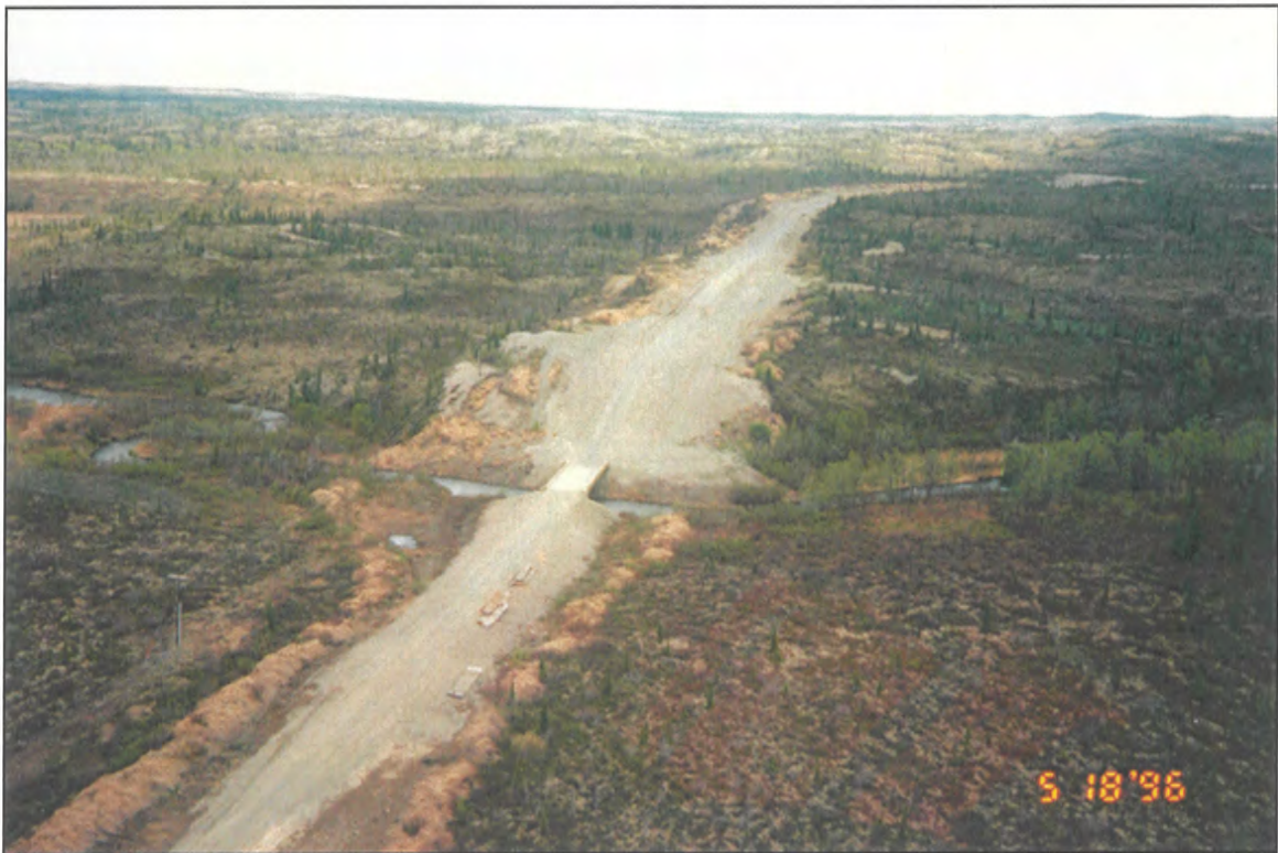
Photo 2: Aerial view of Alexcy Creek Bridge, reconstructed in 1995. 5-18-96.
